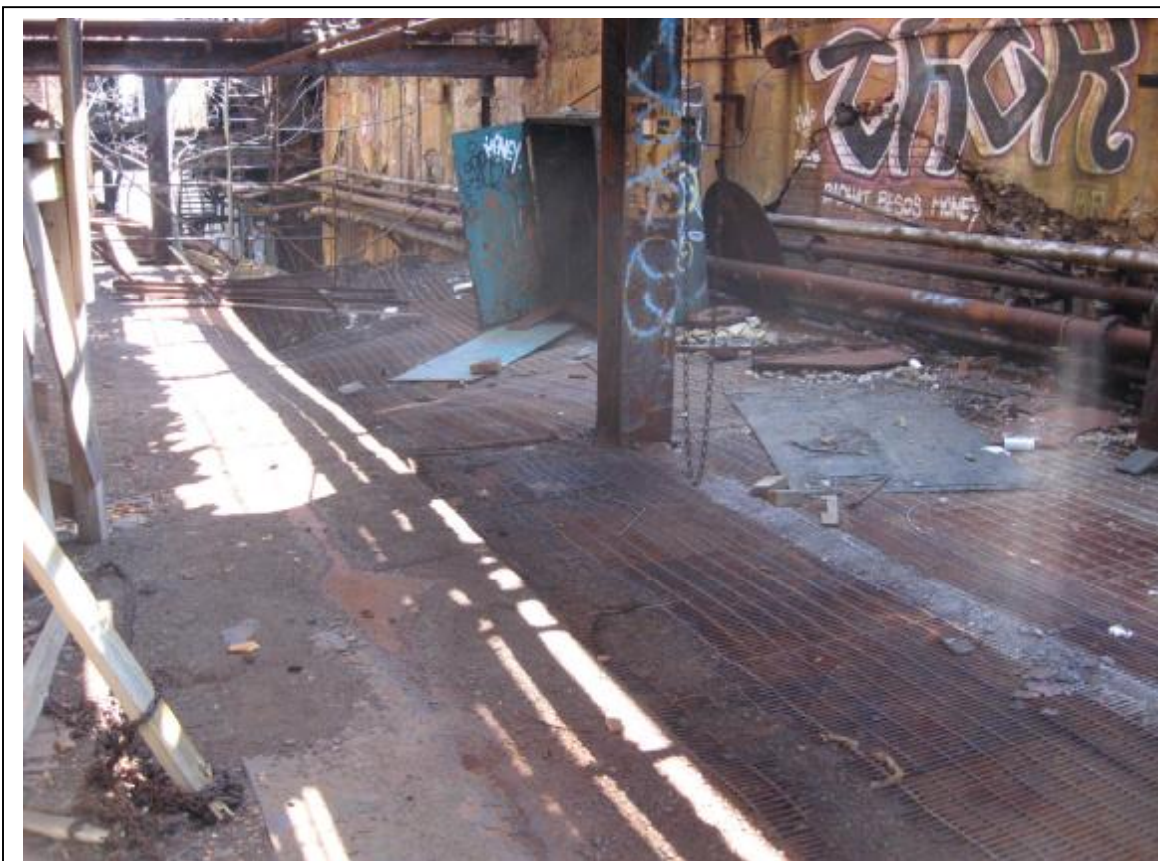
and #2 with critical section loss Photo 62: Walkway between Stoves and Stock House partially collapsed, deformed and settled
