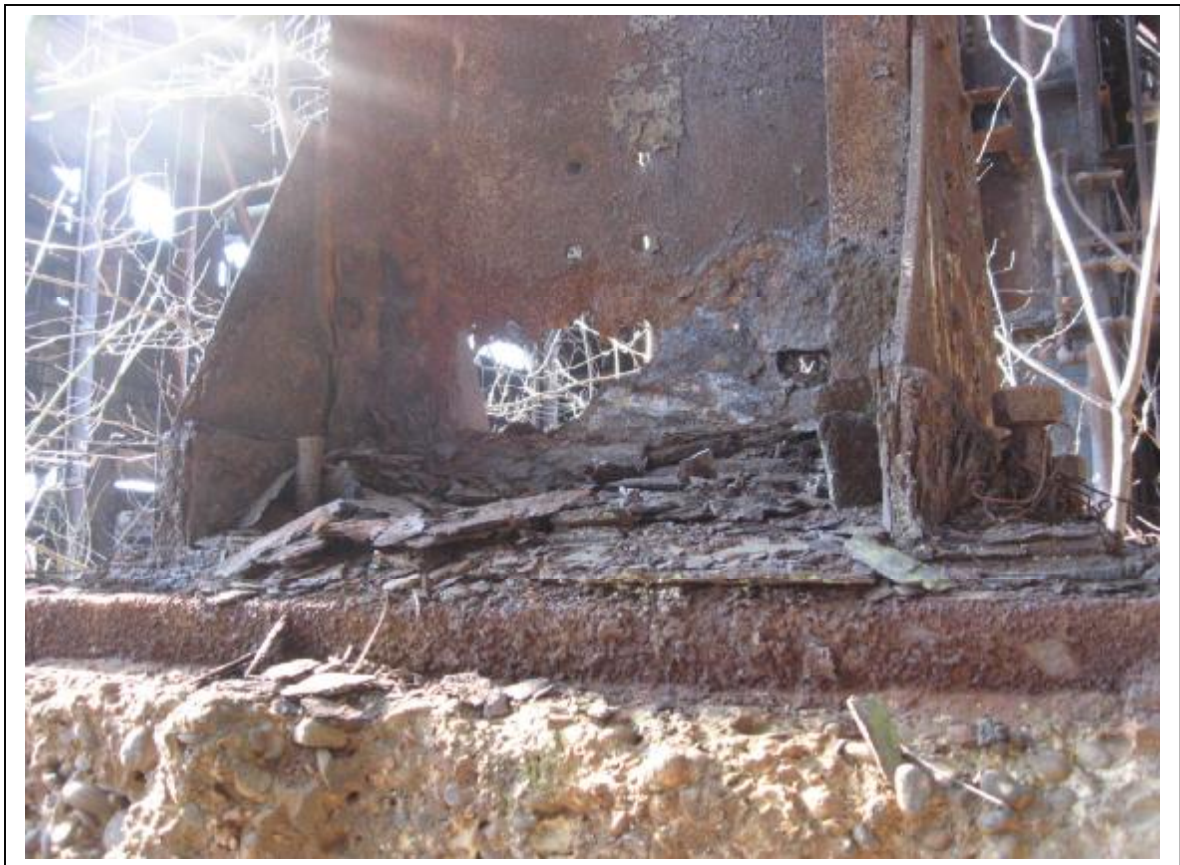
Photo 22: Exterior of Building #2 pipe support member with section loss
