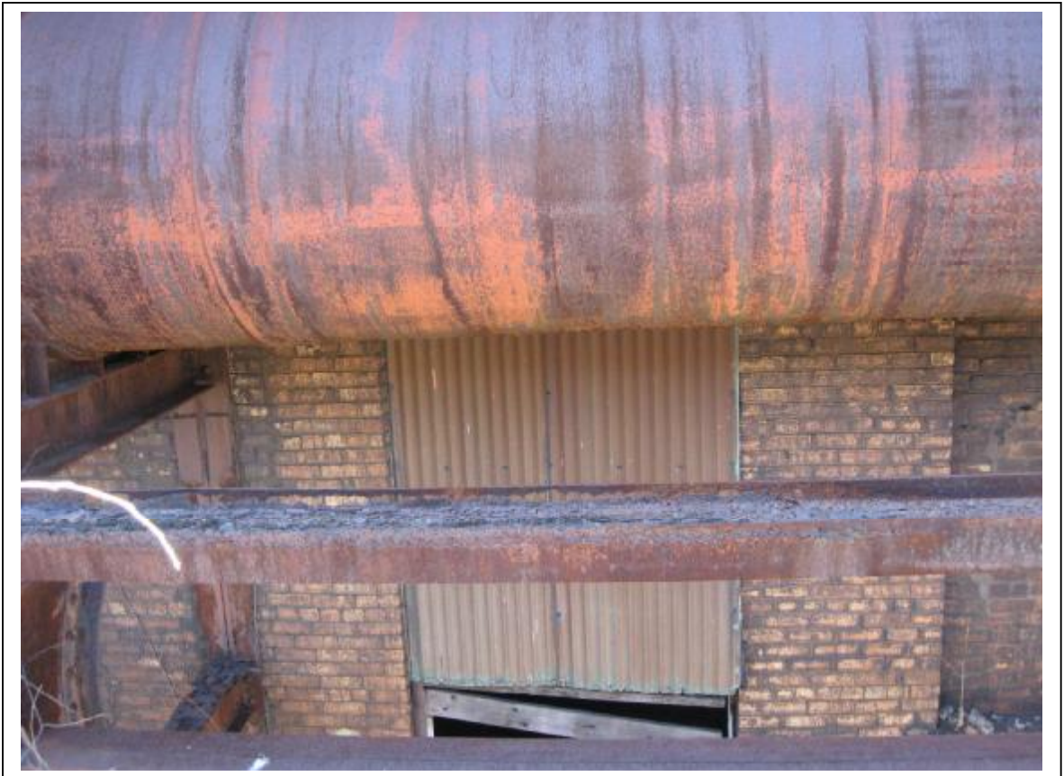
Photo 20: Exterior of Building #2 pipe support with section loss
