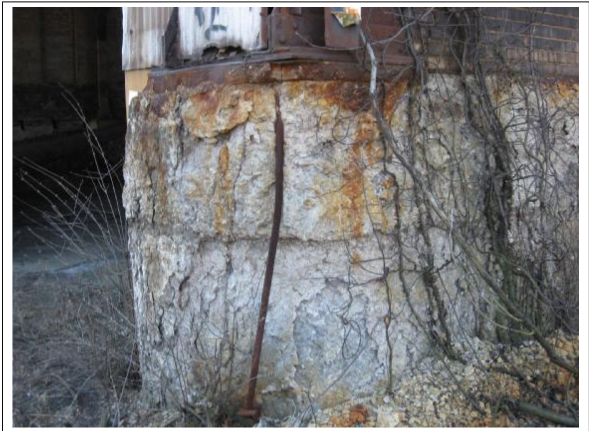
Photo 9: Building #1 Column 1-B anchor bolt completed exposed
