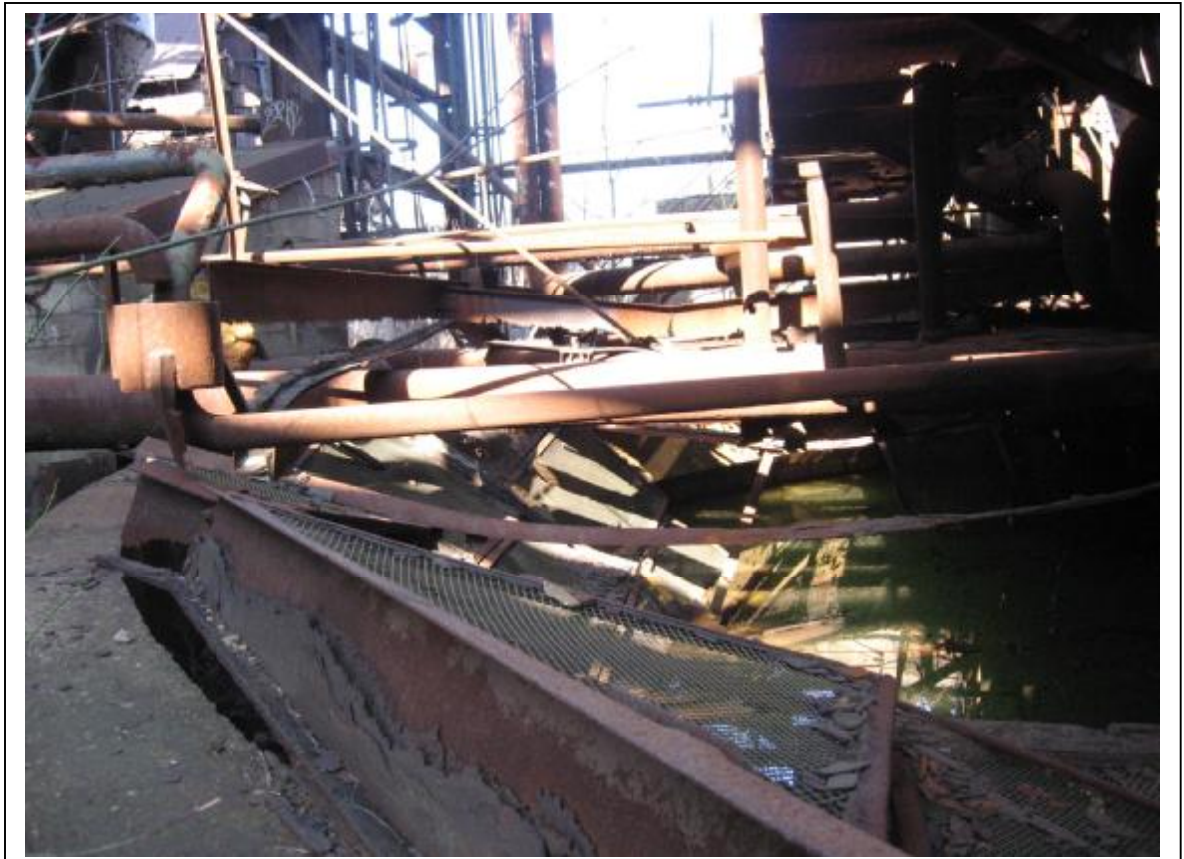
Photo 34: Gas Washers/Electrical Precipitators collapsed and heavily deteriorated members
