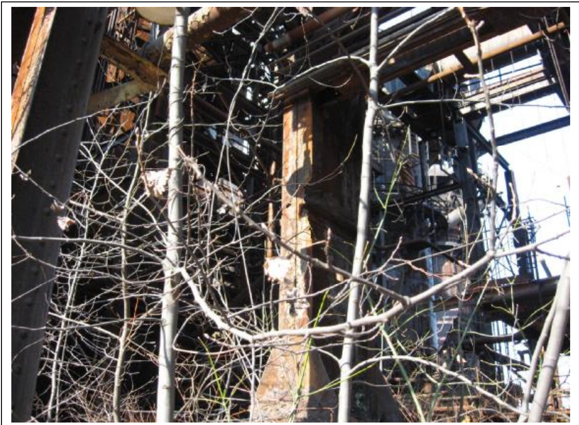
Photo 23: Exterior of Building #2 pipe support member with section loss (roughly 10-ft above ground)
