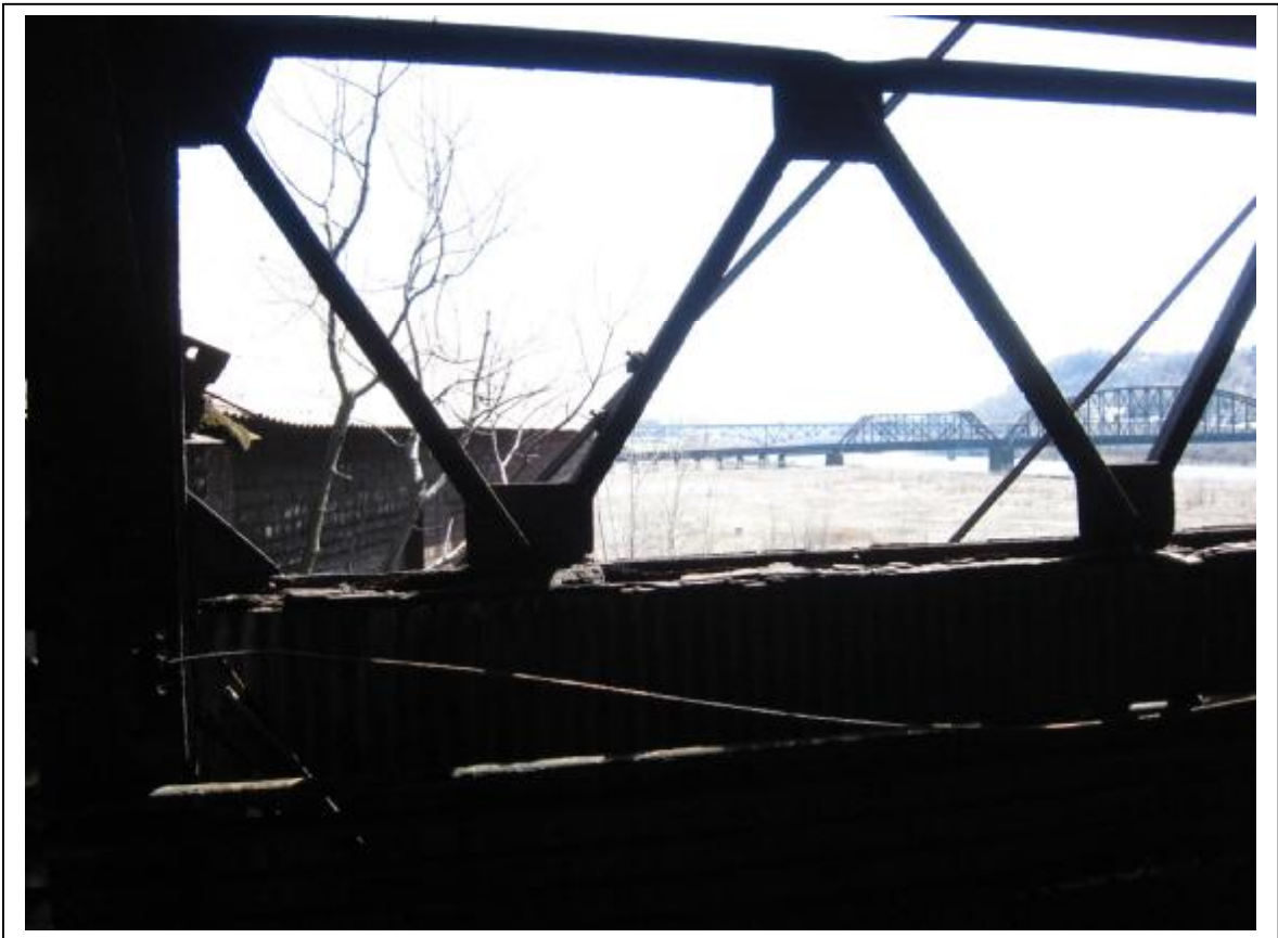
Photo 25: Building #3 roof edge truss on column line A between column lines 3-4 section loss
