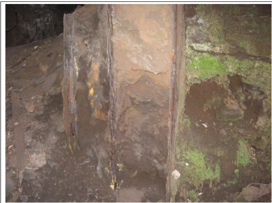
Photo 32: Dust Catcher #2 (North Furnace) Section loss to northern most support column
