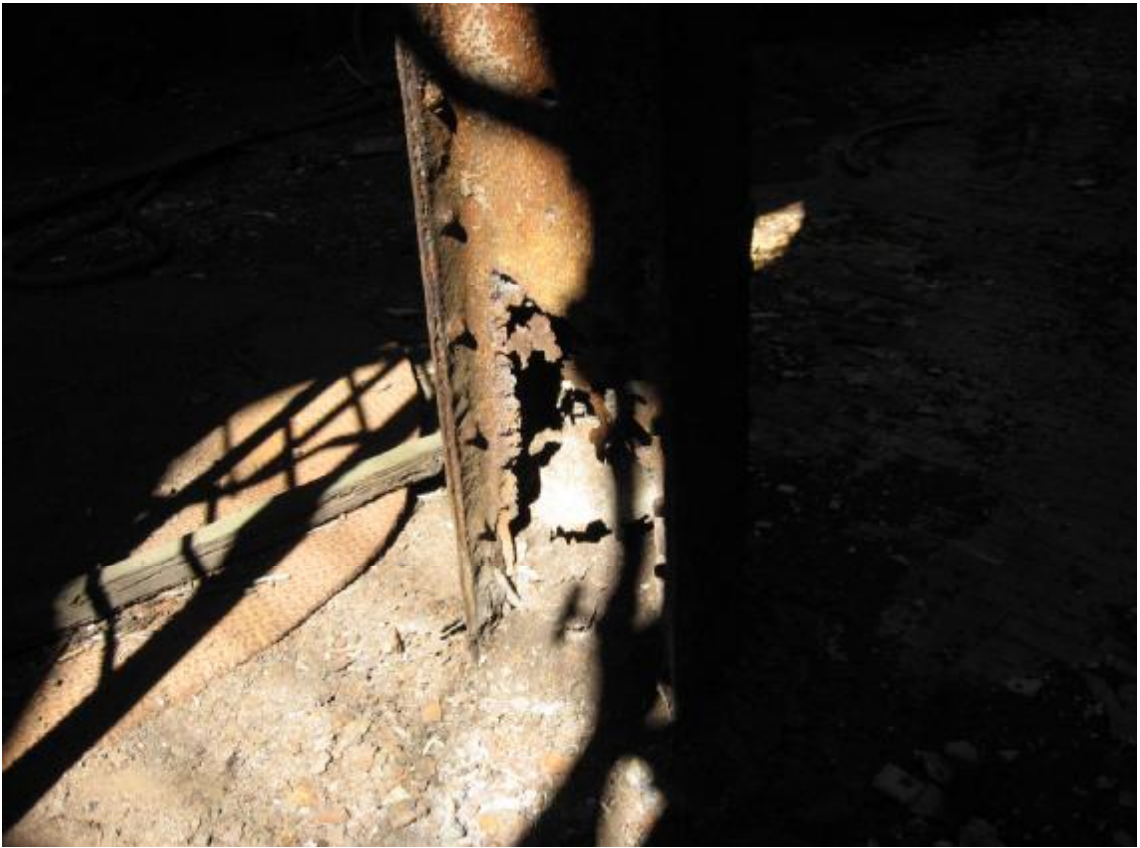
Photo 29: Dust Catcher #1 (South Furnace) 100% deteriorated webs of all four sides of column box
