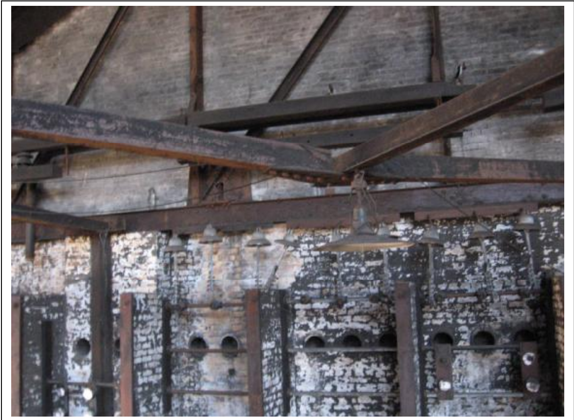
Photo 5: Building #1 missing roof truss lateral bracing
