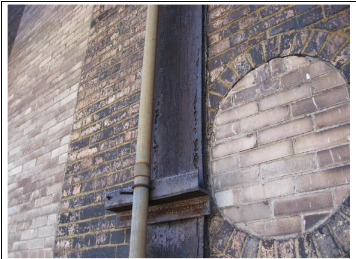
Photo 10: Building #1 Typical condition of exterior column face with section loss to exposed flange
