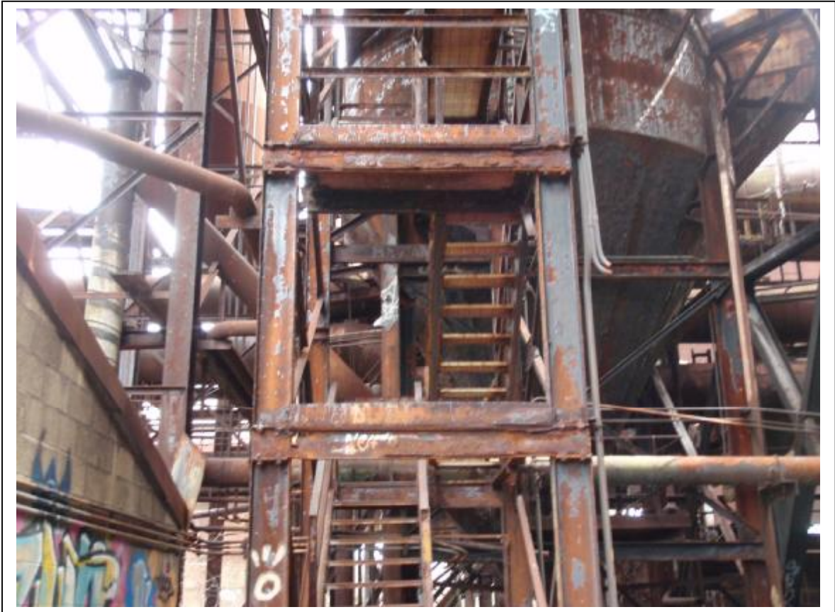
Photo 65: Stair near Electrical Precipitator advanced section loss on members
