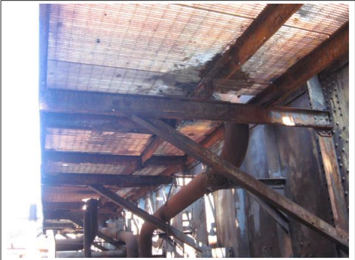
Photo 35: Gas Washers/Electrical Precipitators heavily deteriorated support member for platform
