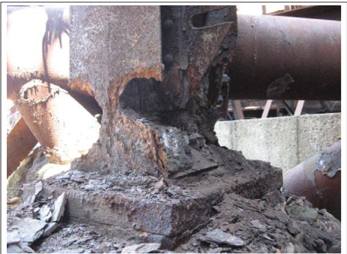
Photo 60: Southern column of tower for pipe support tower between electrical precipitator, and Masonry Building #1 and #2 with critical section loss
