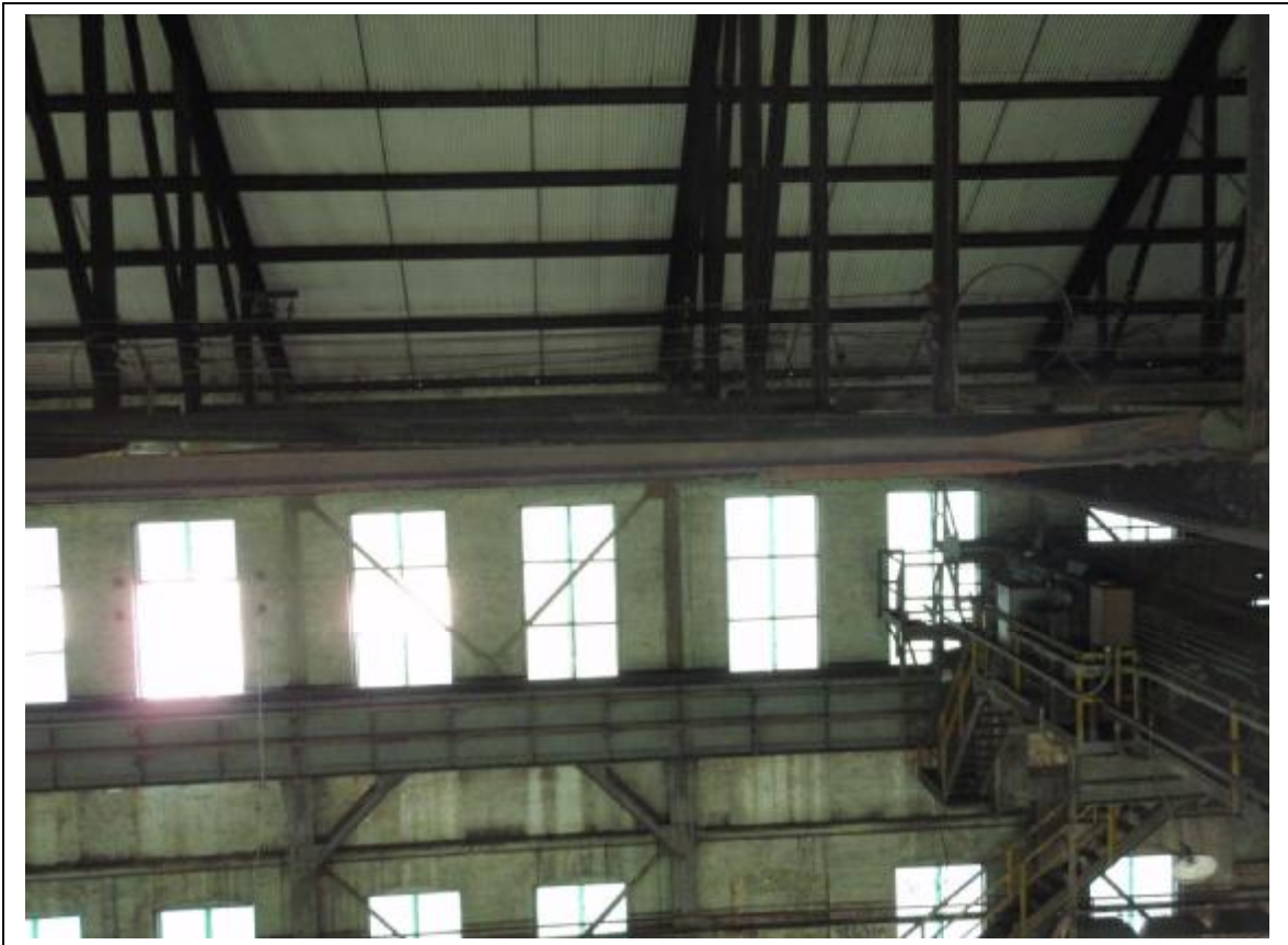
Photo 14: Building #2 twisted lateral bracing of roof truss between columns 3-4 and C-D
