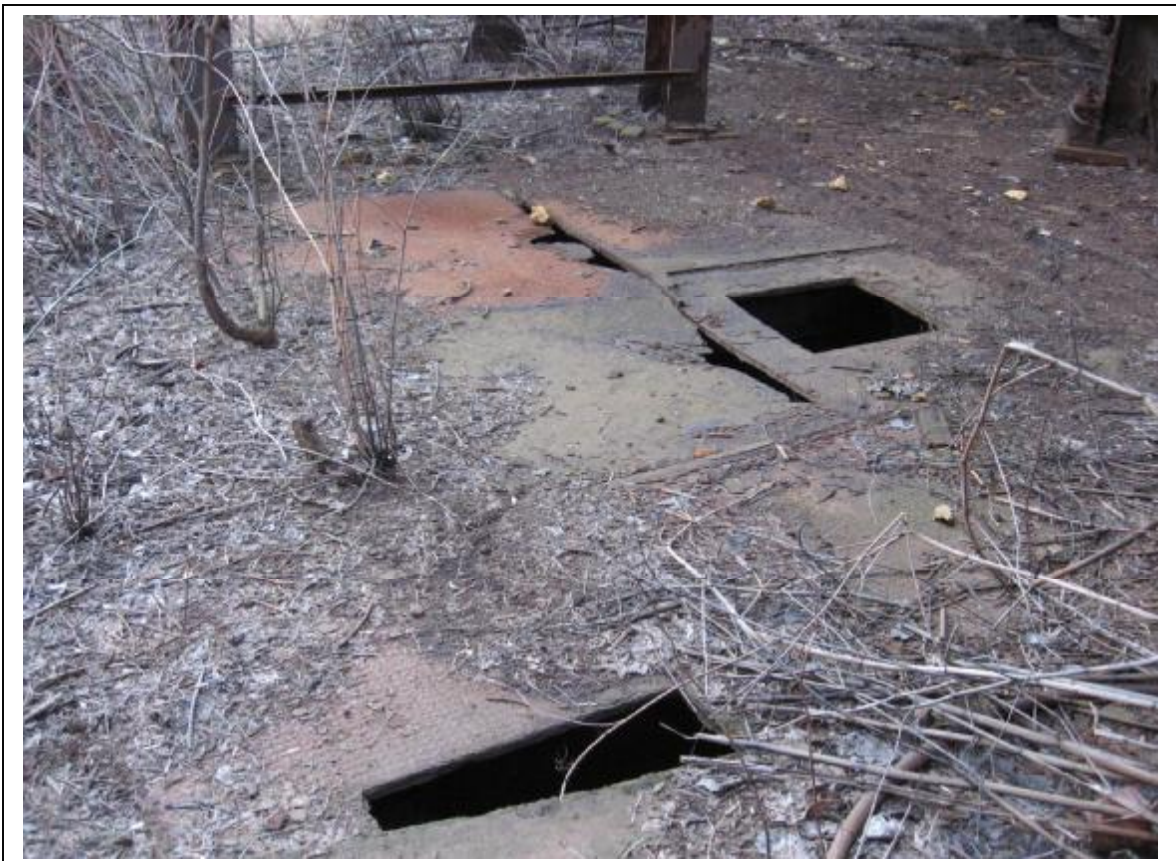
Photo 58: Steel plates covering pit near Masonry Building #1 deterioration
