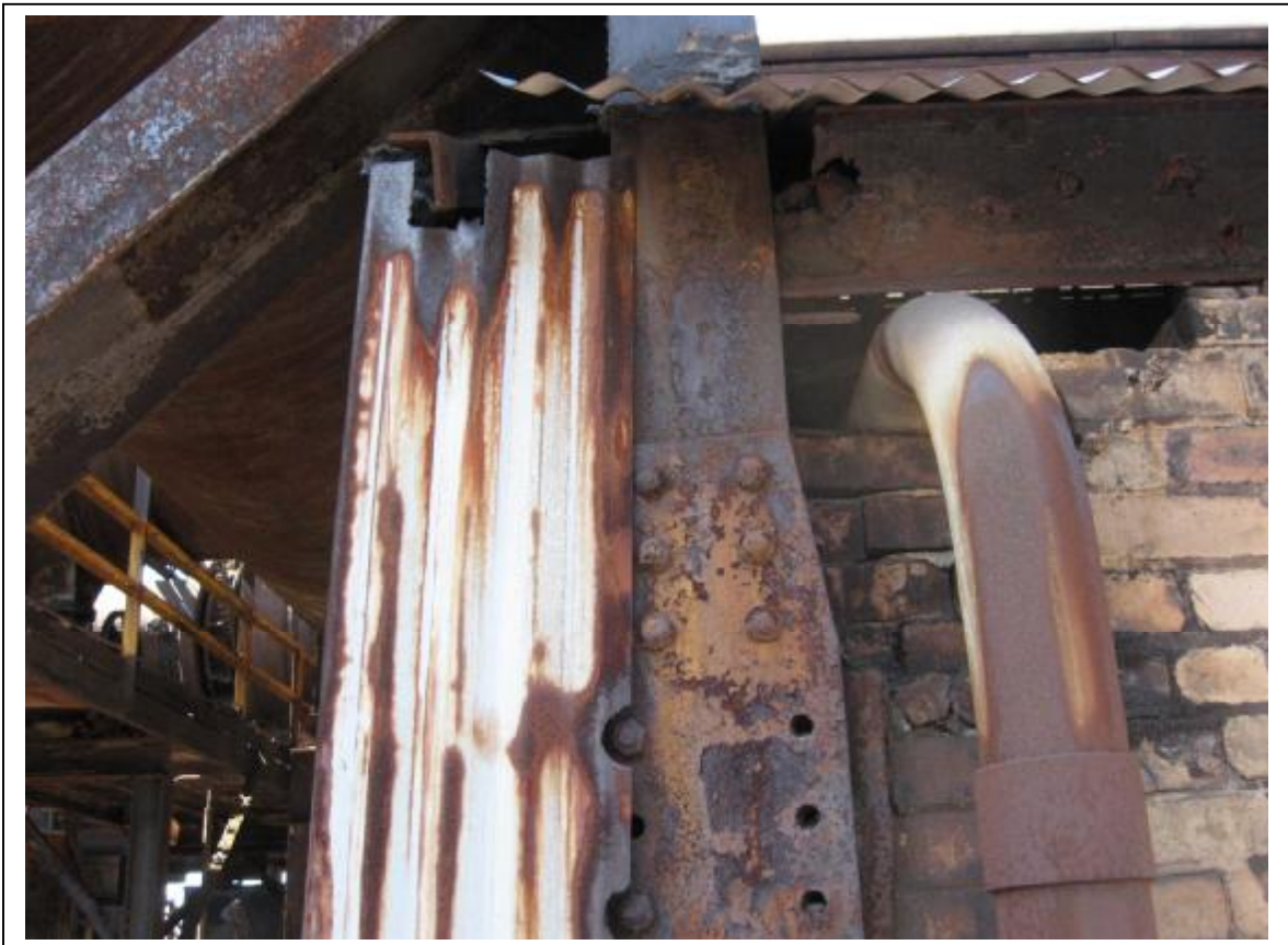
Photo 13: Building #2 Column 12-A near top, four missing rivets
