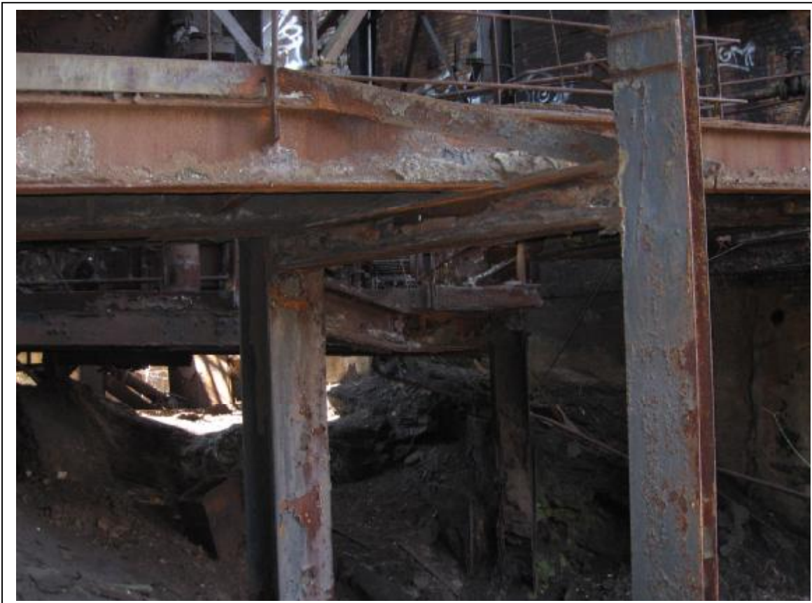
Photo 31: Dust Catcher #2 (North Furnace) Partially collapsed beam and walkway
