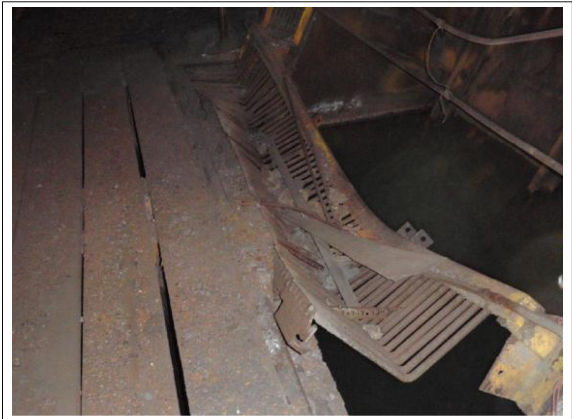
Photo 43: Stock House partially failed bridge at south skip bridge in Stock House
