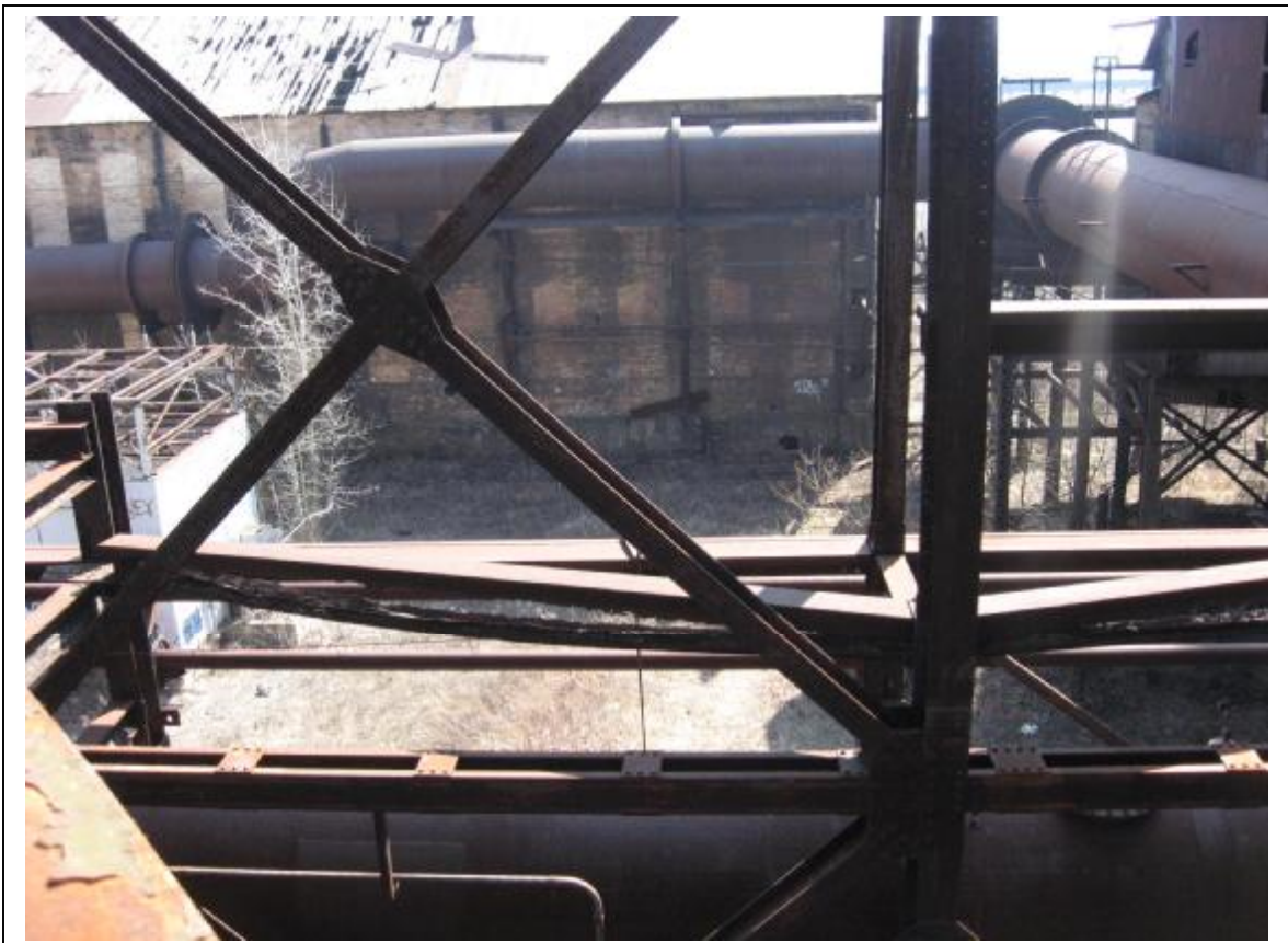
Photo 24: Exterior of Building #2 pipe support lateral bracing member with 100% section loss to webs
