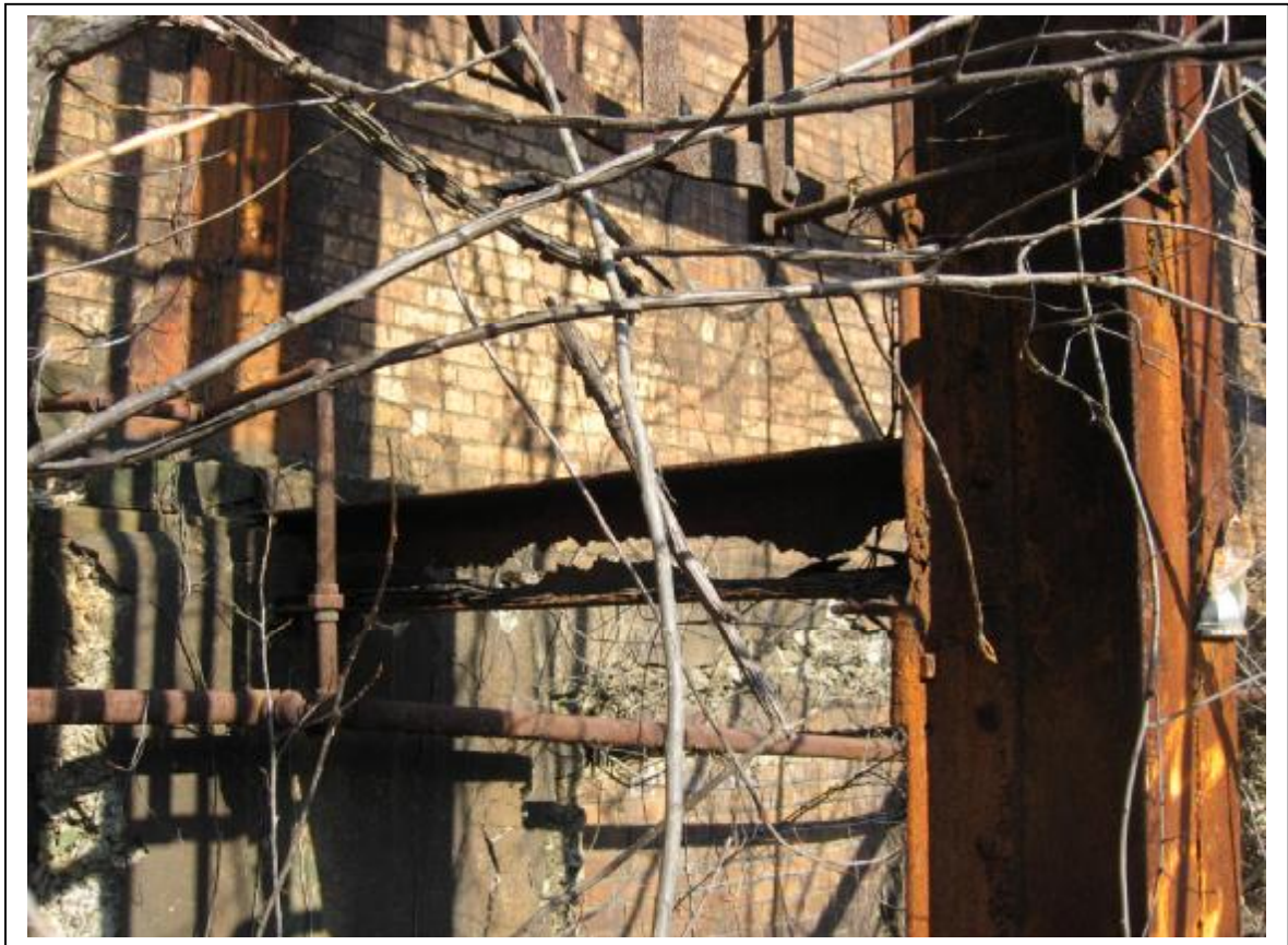
Photo 21: Exterior of Building #2 pipe support member with section loss
