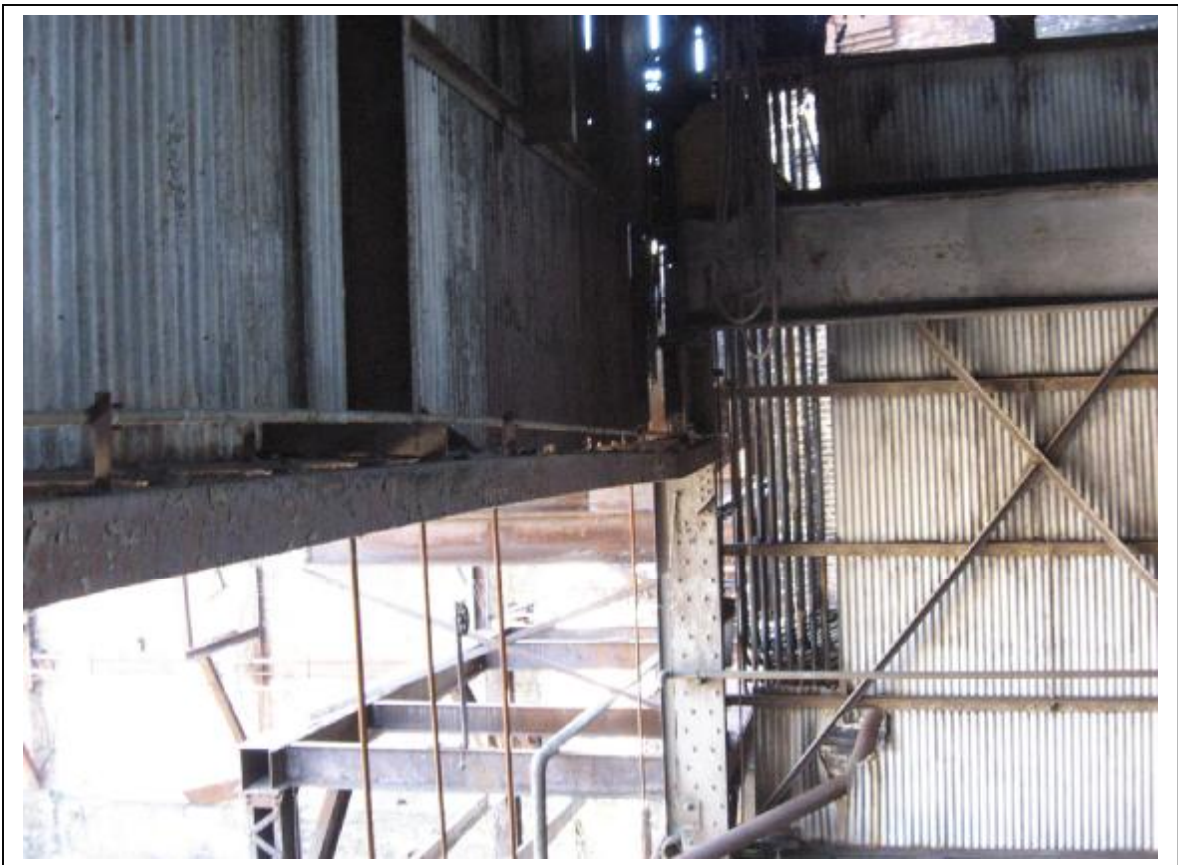
Photo 26: Building #3 deformed edge beam on column line 1
