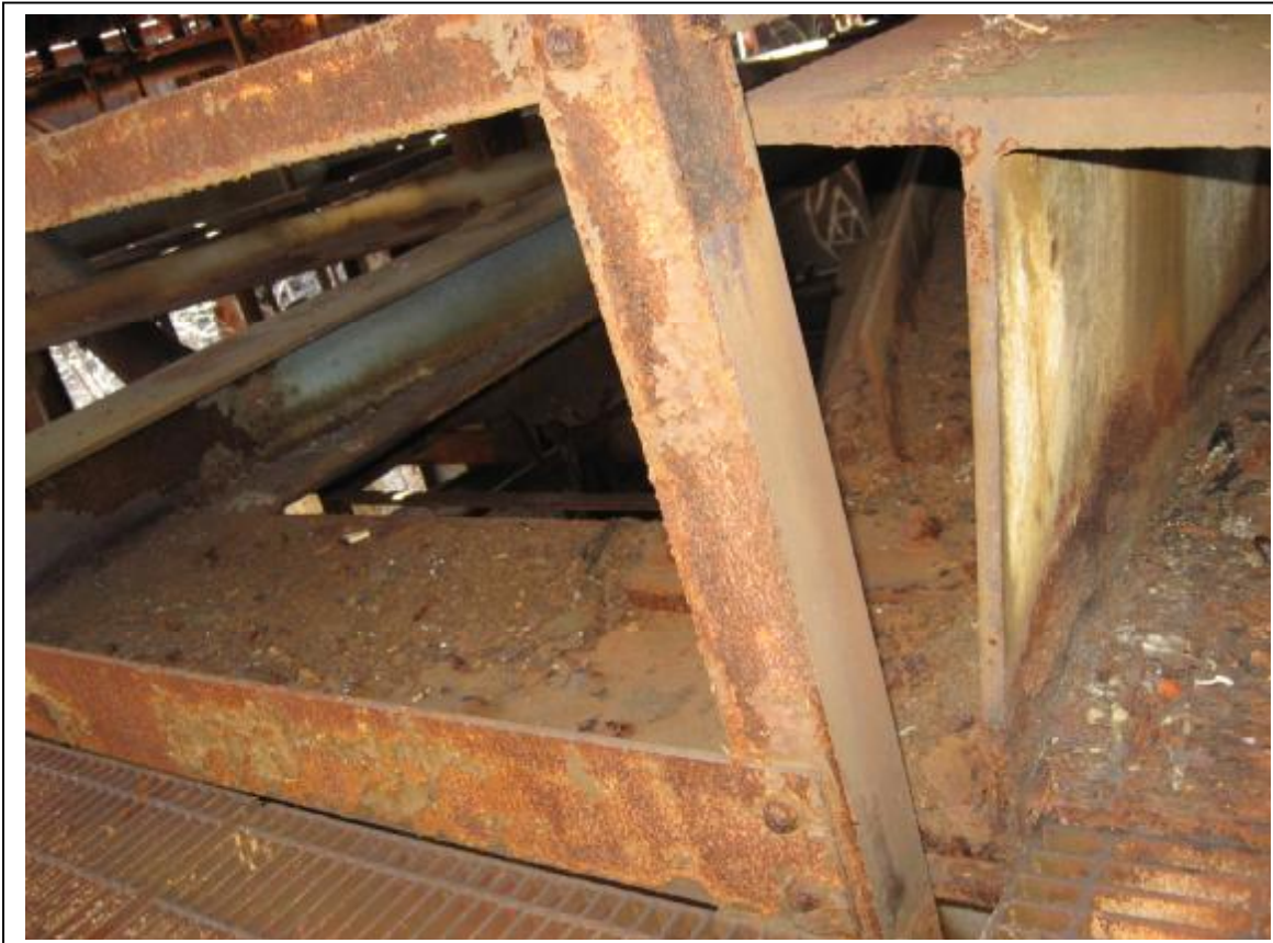
Photo 37: Gas Washers/Electrical Precipitators buckled and rotated support beam located at NE corner of south
