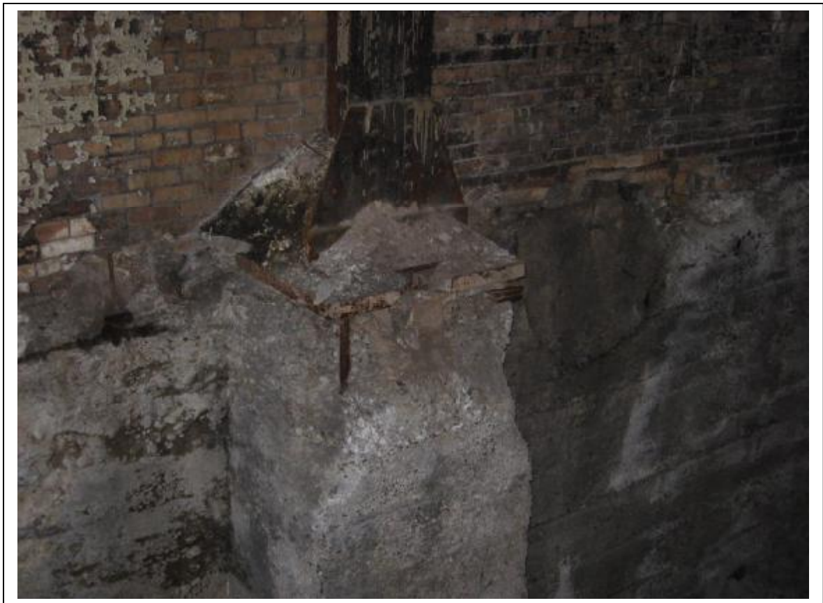
Photo 8: Building #1 Column 17-B, exposed anchor bolts and undermined base plate
