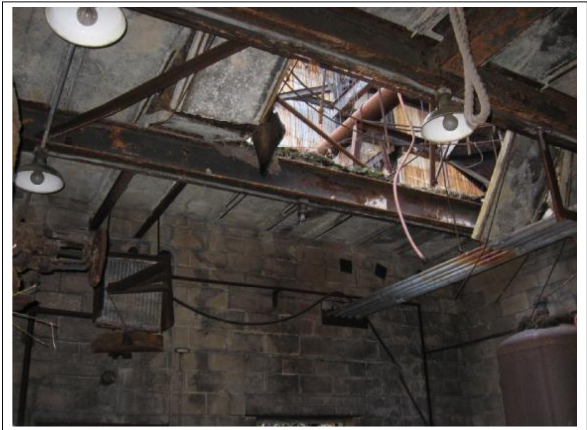
Photo 55: Masonry Building #1 partially collapsed roof and hanging heater unit
