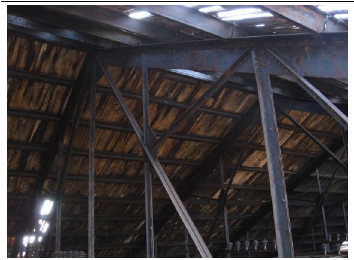
Photo 6: Building #1 Typical roof truss condition
