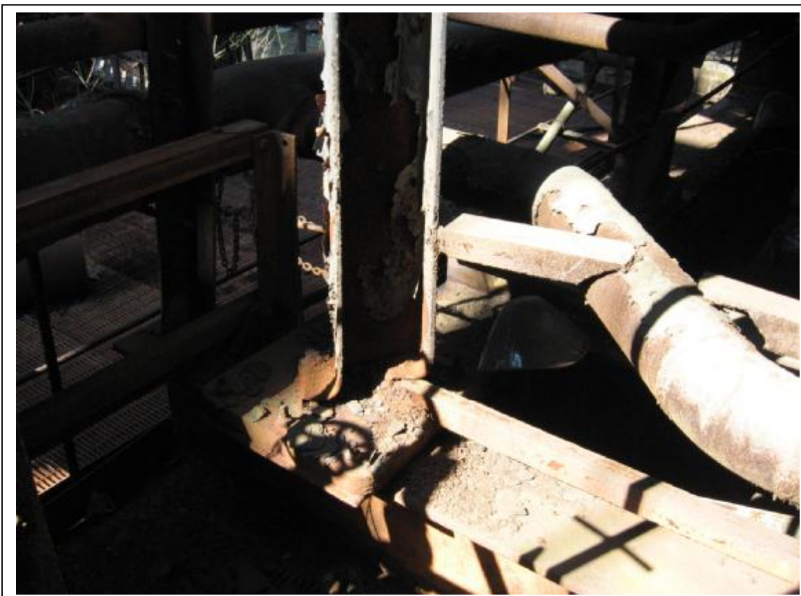
Photo 38: Gas Washers/Electrical Precipitators buckled and advanced deterioration of column that supports the north electrical precipitator
