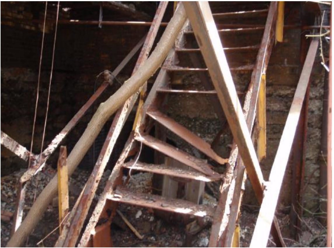
Photo 64: Stairway near north furnace and dust collector collapsed, deformed and settled
