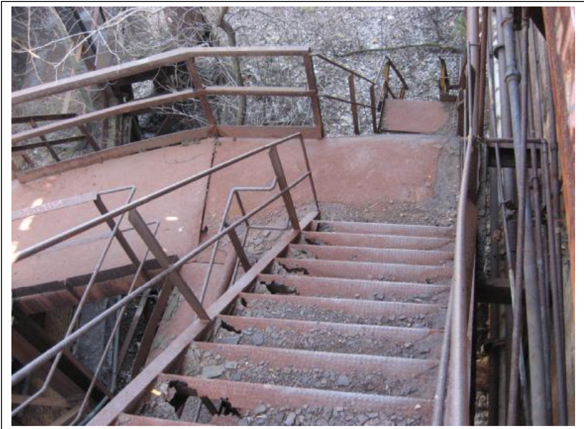
Photo 48: Stair at furnace side of Ore Bridge in unsafe condition
