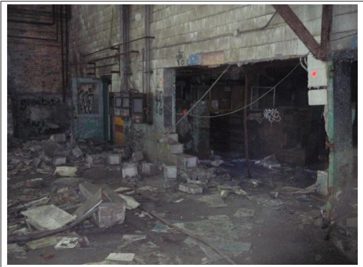
Photo 15: Building #2 Partial demolished office space – “Imminent” failure condition
