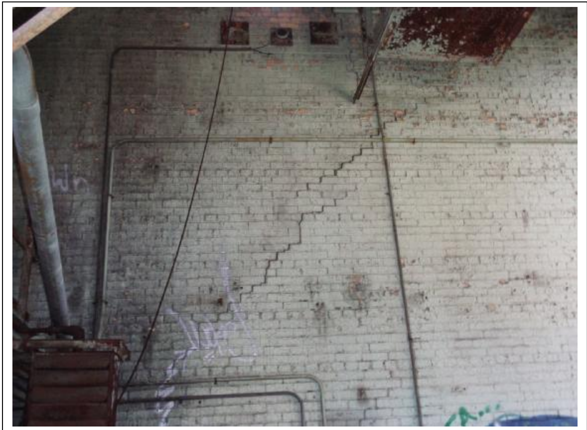
Photo 53: Skip Hoist Motor Building for North Furnace crack in wall
