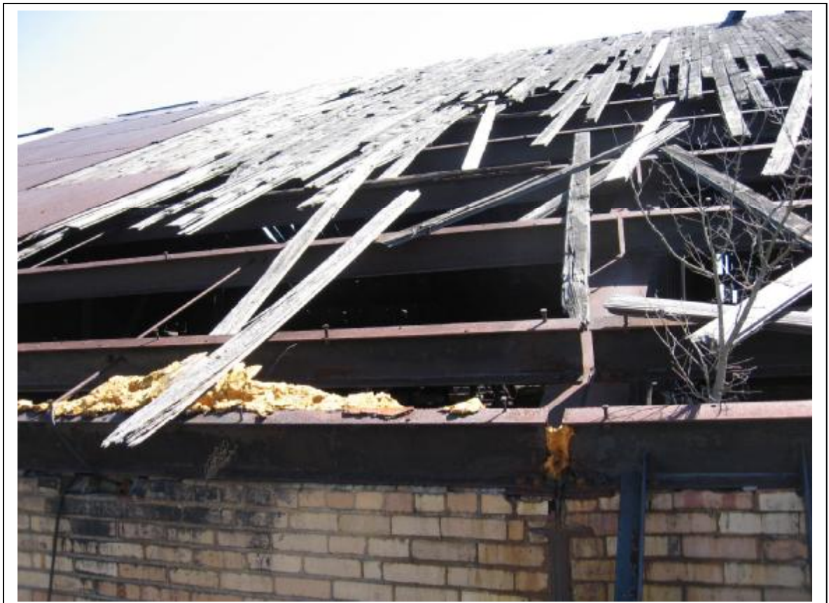
Photo 4: Building #1 with missing and deteriorated roof
