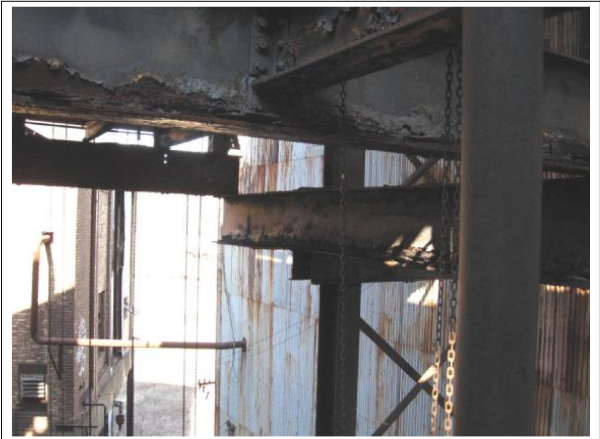
Photo 59: Walkway and pipe support beam between electric precipitators and Building #2 with beam deformation,
