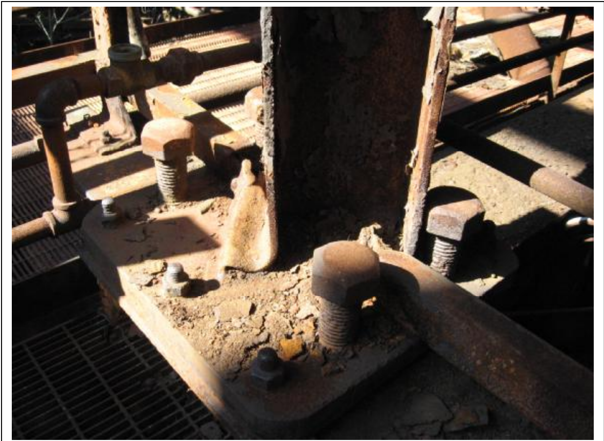
Photo 36: Gas Washers/Electrical Precipitators buckled and advanced deterioration of column that supports the south electrical precipitator
