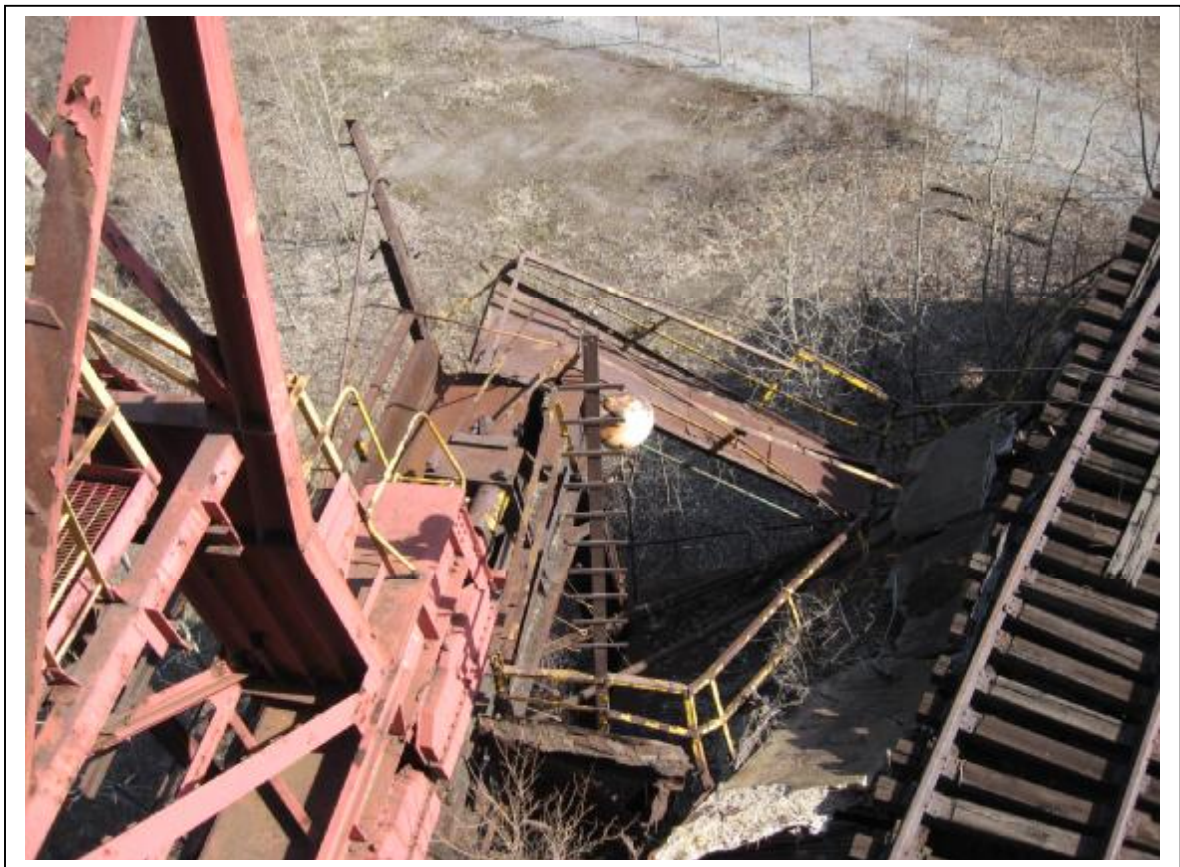
Photo 45: Stock House collapsed walkway at south end of Stock House
