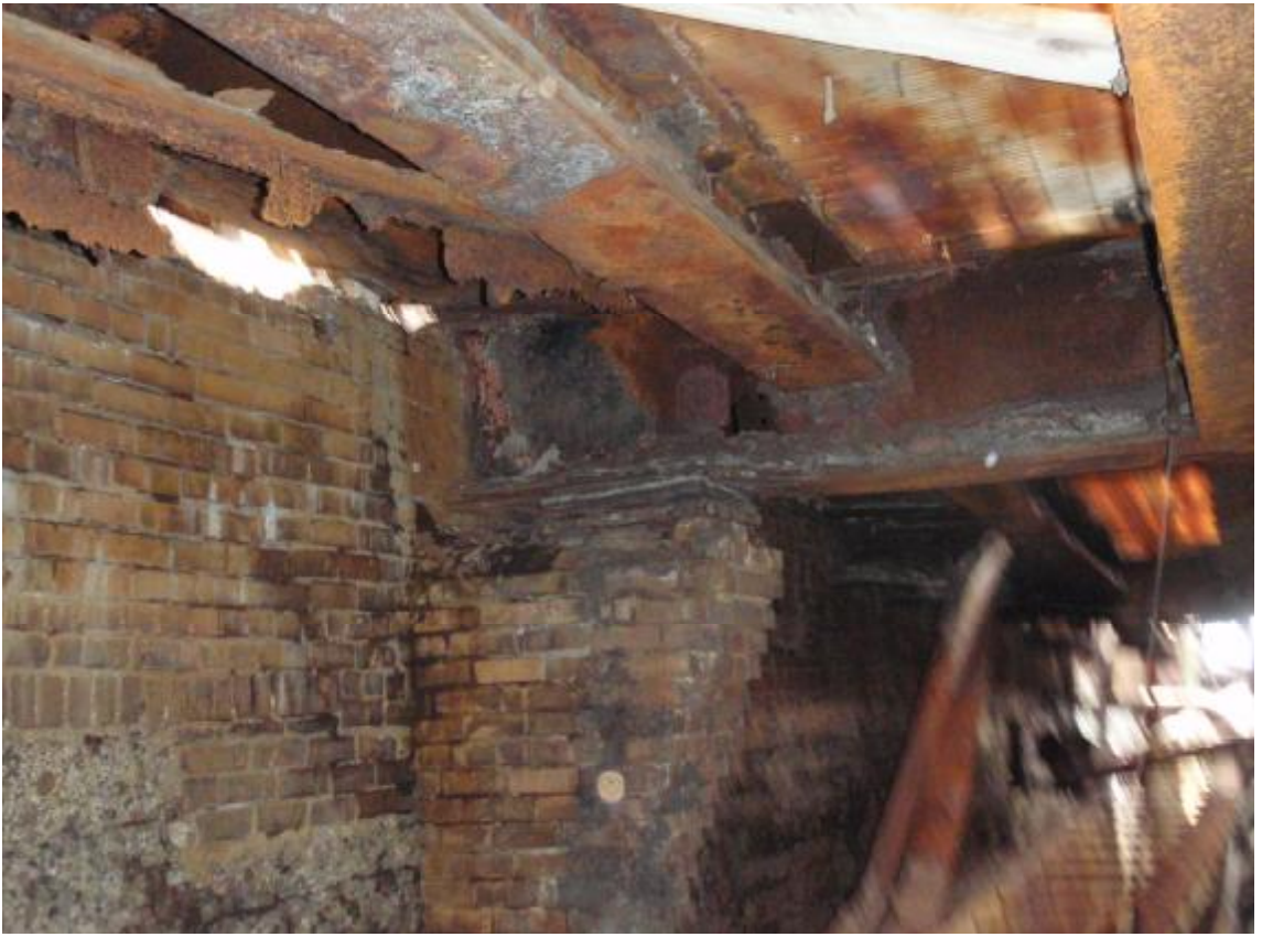
Photo 63: Underside of walkway between Stoves and Stock House partially collapsed, deformed and settled
