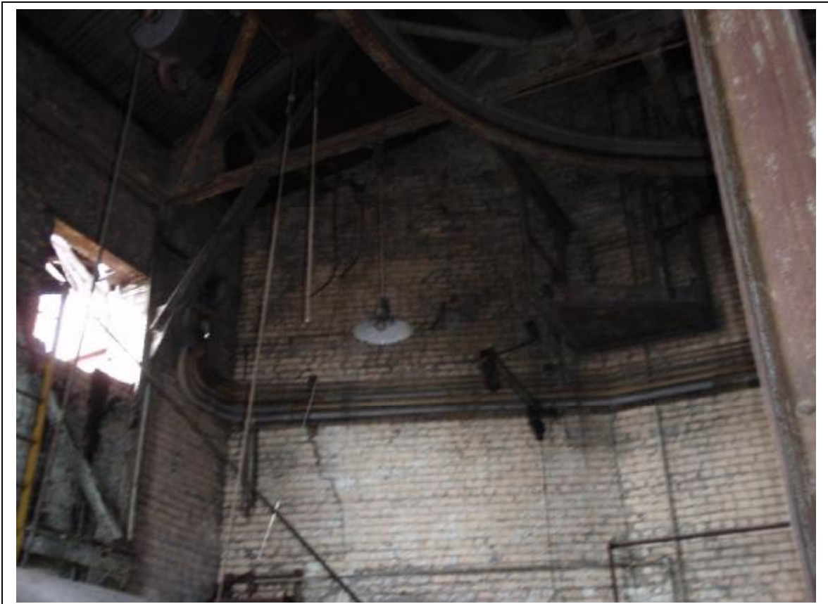
Photo 50: Skip Hoist Motor Building for South Furnace crack in north wall
