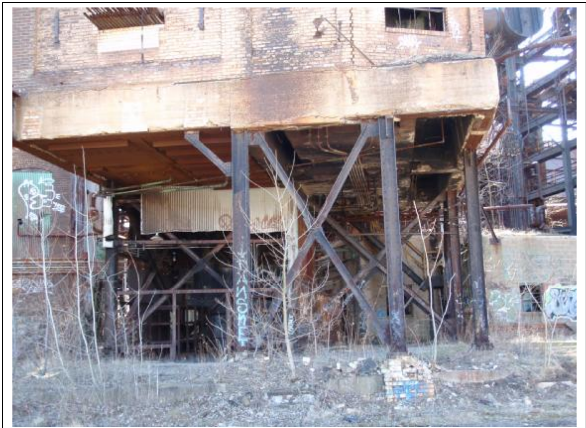
Photo 52: Skip Hoist Motor Building for North Furnace framing underneath it
