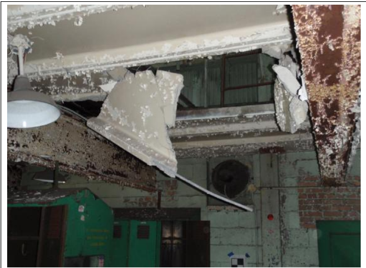
Photo 16: Building #2 Upper floor of office space with roof partially collapsed – “Imminent” failure condition
